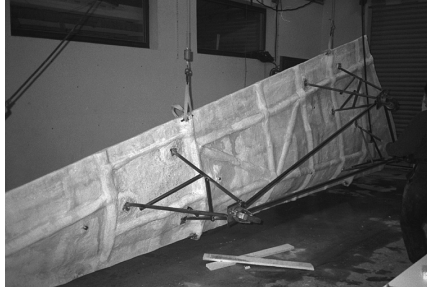
Stiffening ribs of M1 fabric/laminating ceramic reinforce the rear side of the mould
